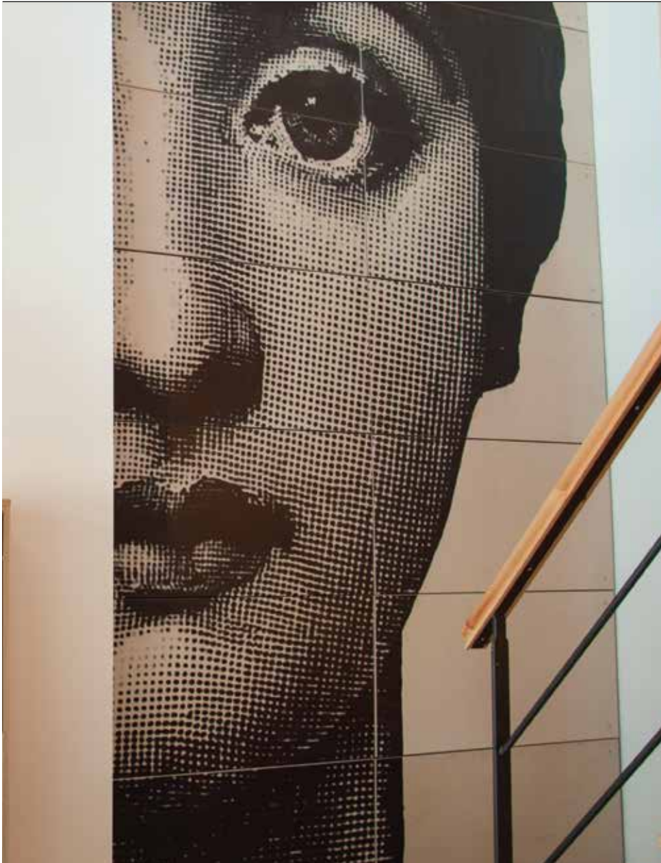
GRC printed indoor façade panels Project: Loft Suite Project, Limassol, Cyprus
