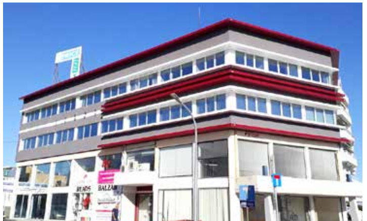
Installation and supply of special façade for residential building at Limassol, Cyprus / perforated honeycomb panel with concrete surface (Cyfield)
