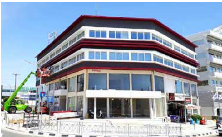
Installation and supply of louver made of aluminium honey comb and aluminium surface for commercial building at Limassol, Cyprus
