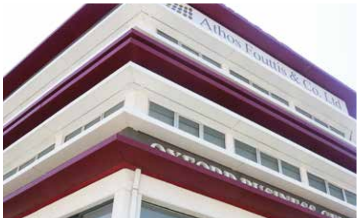
Installation and supply of louver made of aluminium honey comb and aluminium surface for commercial building at Limassol, Cyprus
