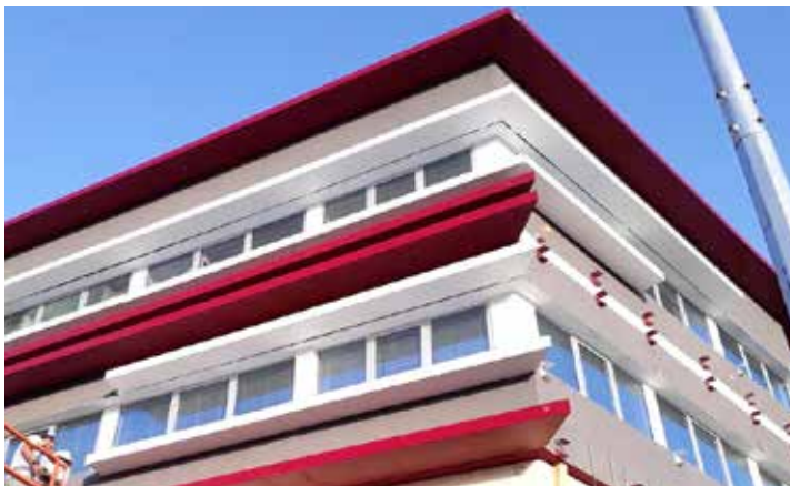
Installation and supply of special façade for residential building at Limassol, Cyprus / perforated honeycomb panel with concrete surface (Cyfield)
